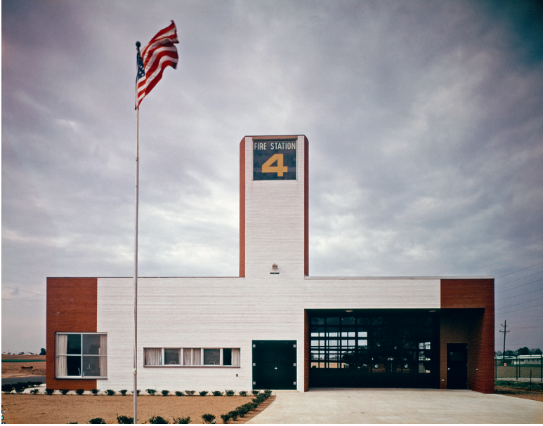
FIG. 9 Fire Station Number 4, Columbus, Indiana, designed by VSBA.
